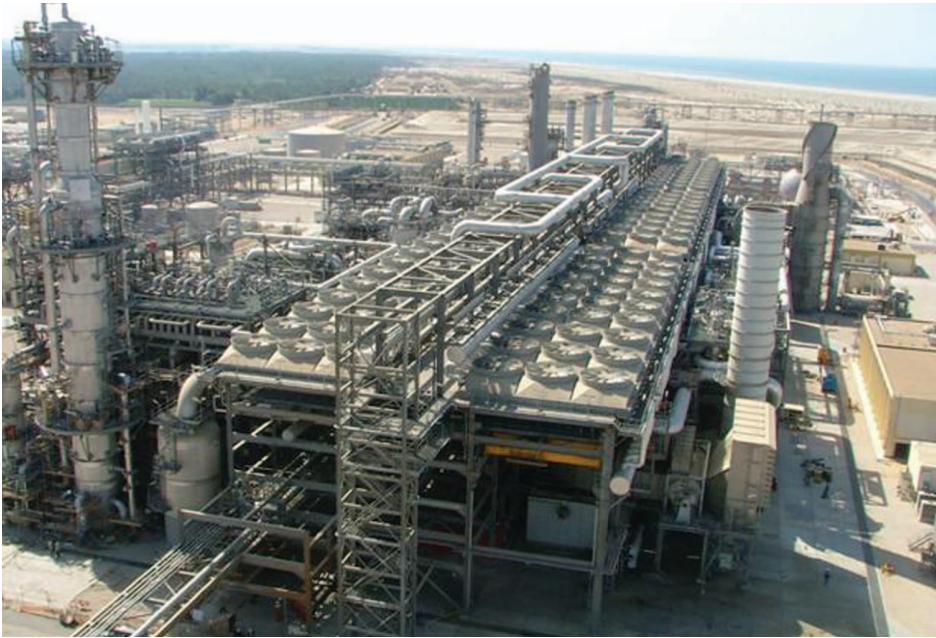
Natural Gas Liquefaction Facility. (Picture Courtesy of Segas)
